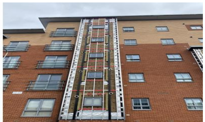
B3 Now Ready For Fire Stop & Insulation
